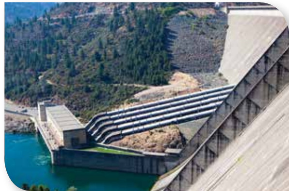
HYDROPOWER PLANT, SHASTA DAM
