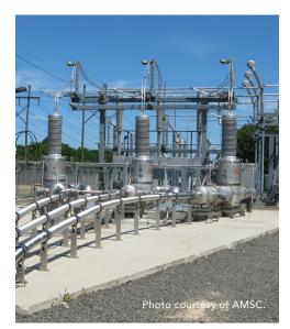
Long Island Power Authority (LIPA) is utilizing a cable system manufactured by Nexans that utilizes AMSC's HTS wire and an Air Liquide cooling system. Energized in April of 2008, this is the world's first superconductor transmission-voltage cable system and is capable of transmitting up to 574 megawatts (MW) of electricity and powering 300,000 homes.
